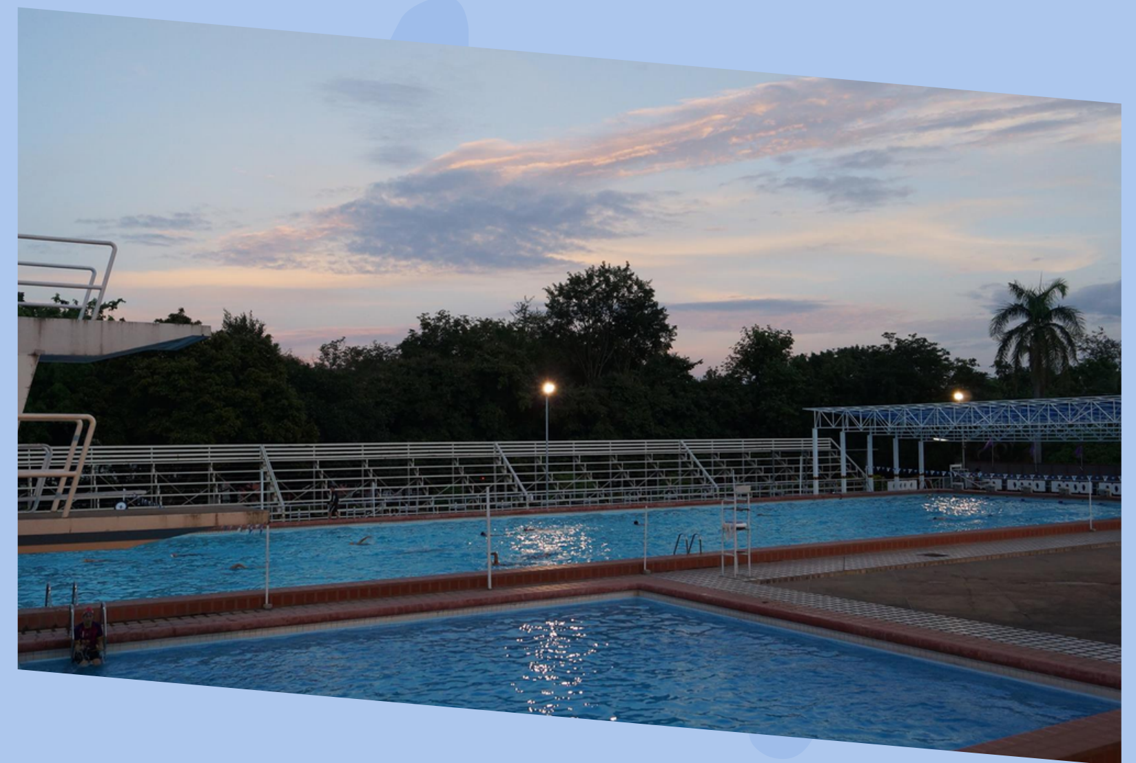
Rujirawong Swimming pool
